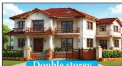
Double storey house
