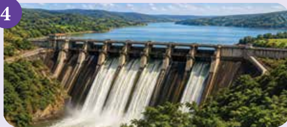
Tehri Dam Project (Uttarakhand)
