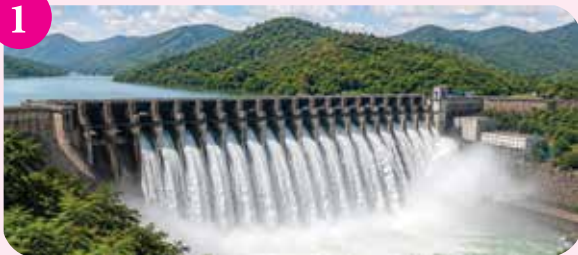
Tehri Dam Project (Uttarakhand)
