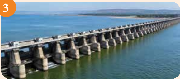
Tehri Dam Project (Uttarakhand)
